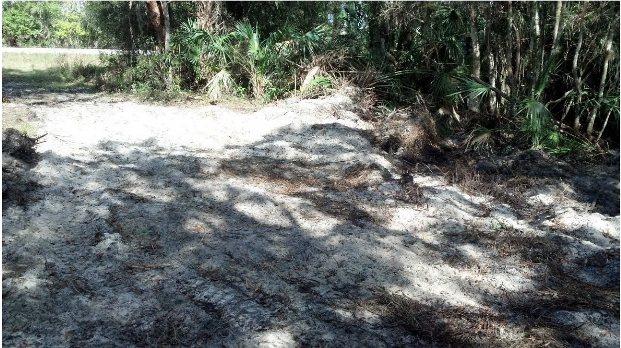
The channel of Cowpen Slough filled on the south side of Fruitville road. Fruitville Road is in the background. It appears as this may be an attempt to construct a crossing form livestock and agricultural vehicles.
