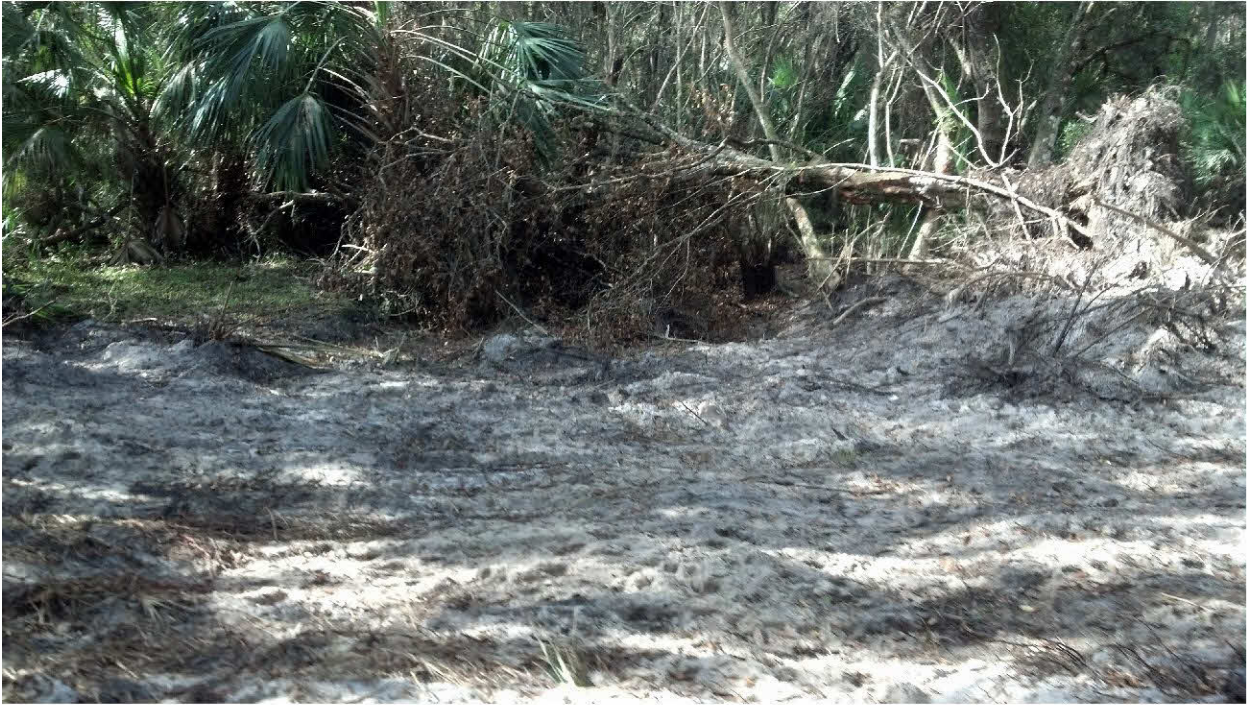
Clearing and filling of the Cowpen Slough Channel.
