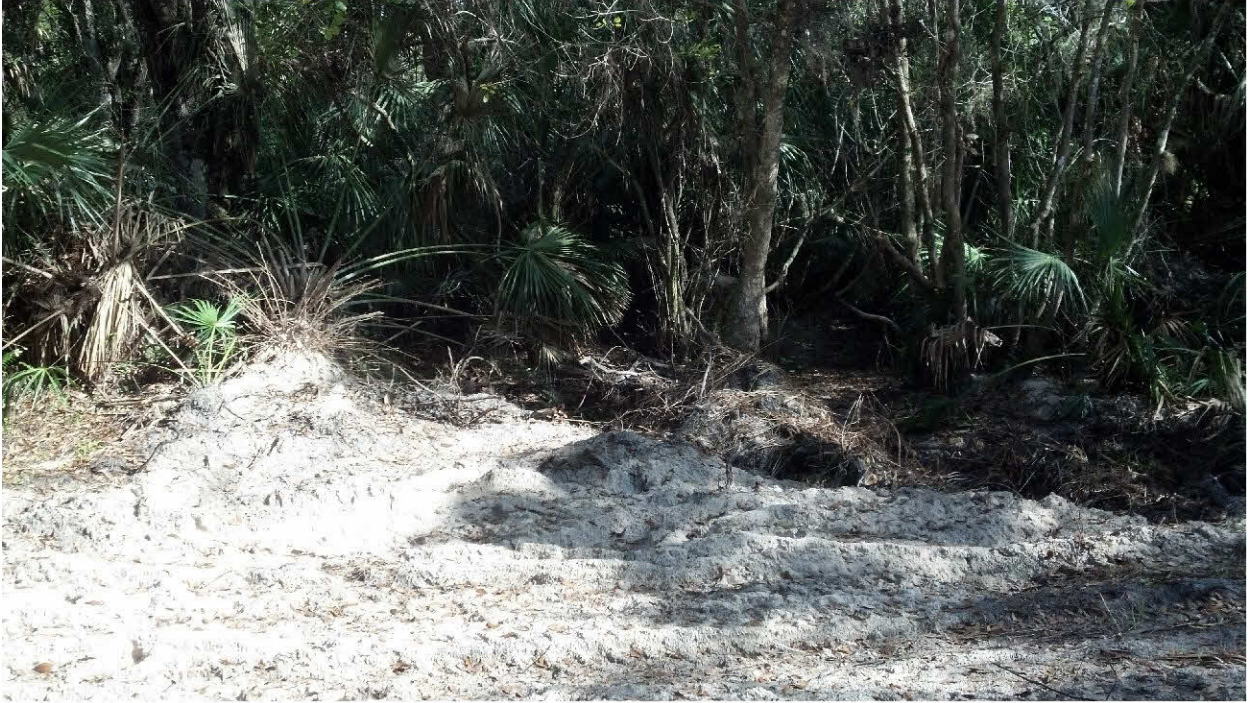
Clearing and filling of the Cowpen Slough Channel.
